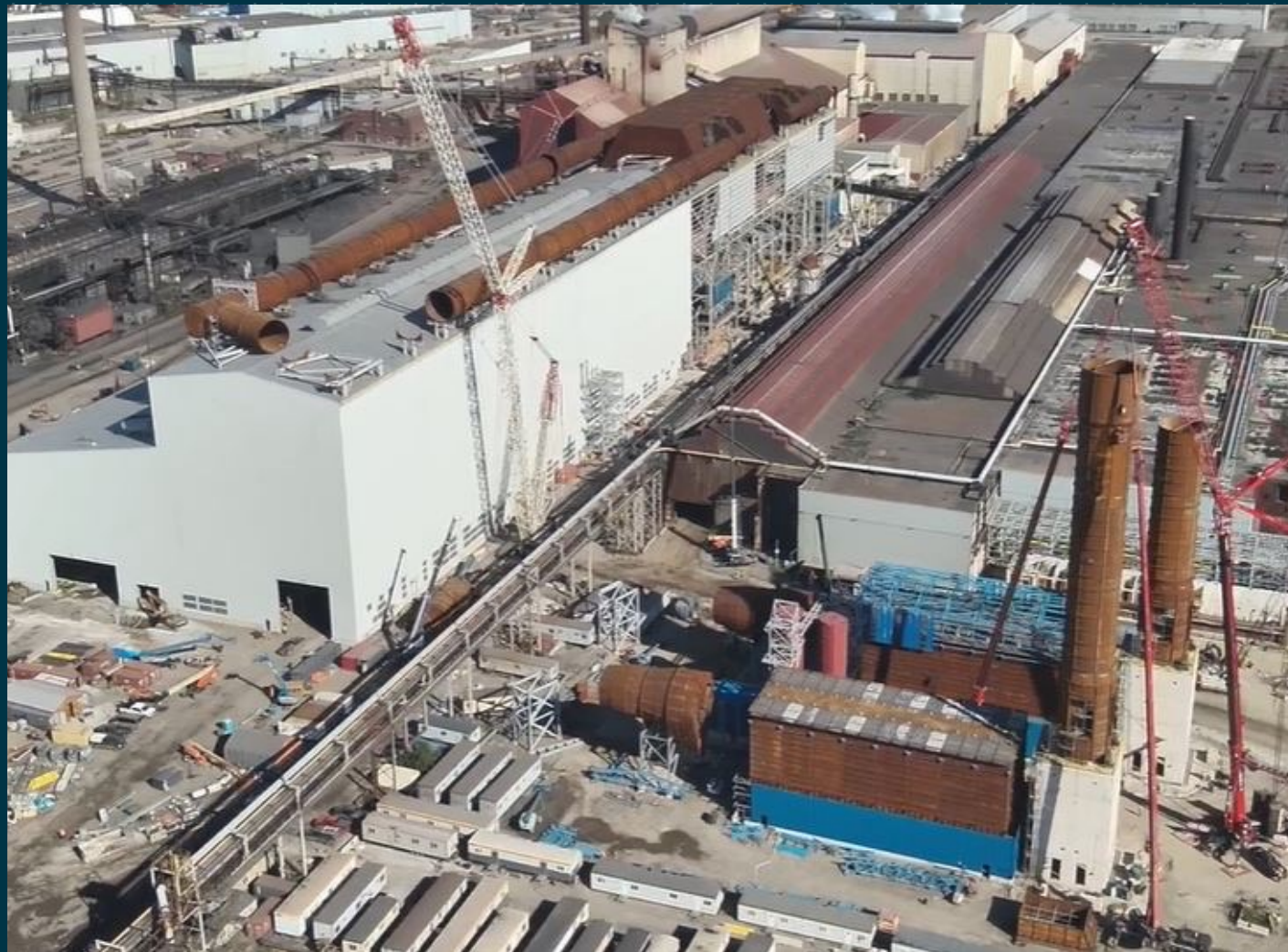
Stacks on Fume Treatment Plant (FTP) installation
